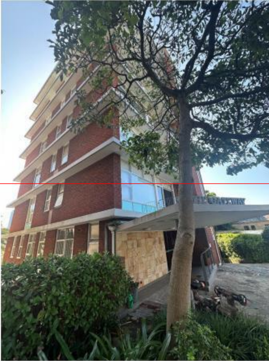
Figure 4. Gateway, 3 Wylde Street. Source: GML Heritage, 2024.
